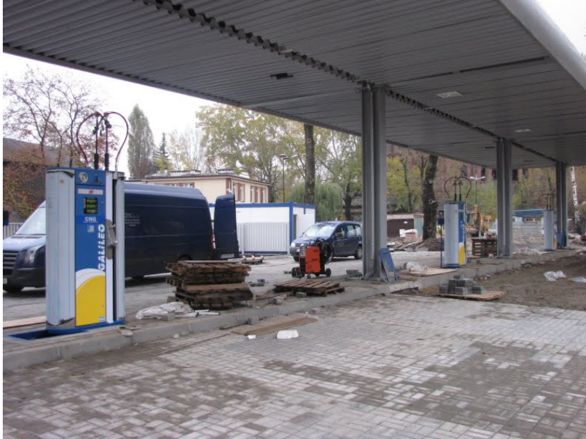
Picture 4 Gas filling station at Prądzyńskiego St. in construction phase
